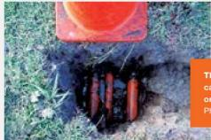
TIP: Physically locate underground electrical cables by pot-holing using hydro-excavation or other non-destructive digging techniques. Photo: IPWEA Australasia
